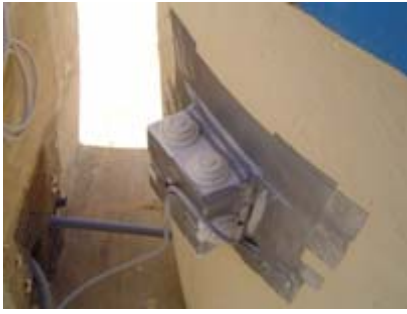
Figure 7: The capacitive sensor used to control tank level
