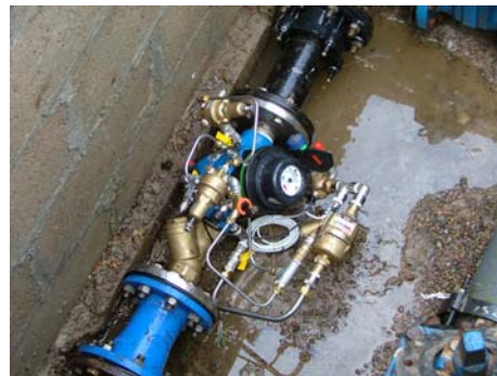
Figure 17 Installation of the hydrometer for Flow and Pressure Control system (FPCV)
