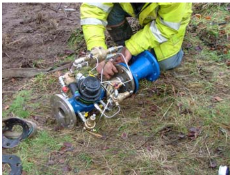
Figure 17 Installation of the hydrometer for Flow and Pressure Control system (FPCV)
